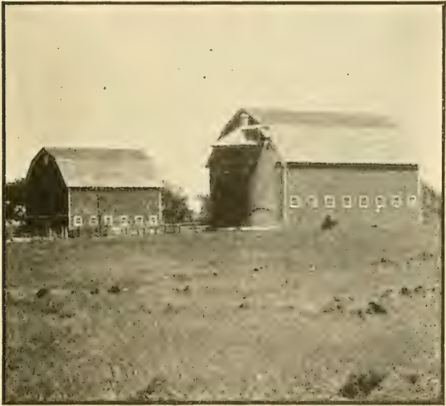
Fig 36—Silo Attached to Barn
